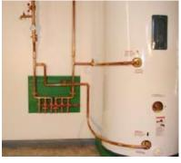
Note: Plan to avoid over heating at plastic fittings. The solar collector antifreeze loop can get very hot if it is only making domestic hot water. Make sure that heat cannot conduct to plastic fittings or other components that are not rated for high heat. The tubing that connects to the solar domestic tank can get very hot. Provide 18 inches of uninsulated vertical separation between the solar tubing and any plastic connections at the supplements manifold.
