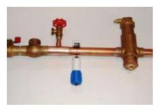
■ Cut the tubing where indicated and attach elbow fittings (not supplied).
