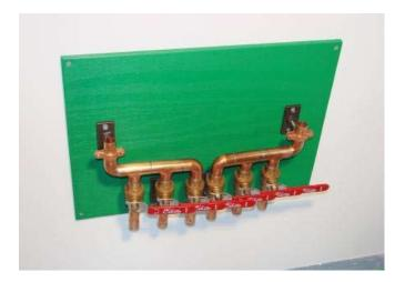
■ Use threaded rod hangers to support the manifold and provide clearance for pipe insulation.
