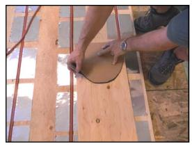
Take this piece of cardboard and place it down on a piece of plywood and trace it. Take a jig saw and cut around the half moon. Now take this piece of plywood and put it back in place on the inside of the tubing bend. To fill in the corners, follow the pictures below.
