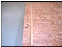
Using a piece of the ¾" plywood for a spacer, screw the strips down leaving a ¾" gap between them. At the end of the run where the tubing will turn 180 degrees, end the plywood strip about 12" away from the picture frame. This will allow for the tubing to bend and you'll fill in this area during a later step.
