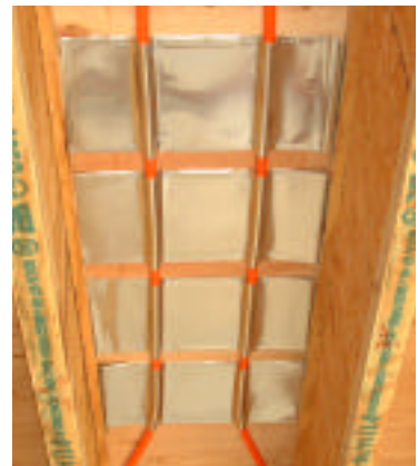
Two tubes per joist, 1/2" PEX
