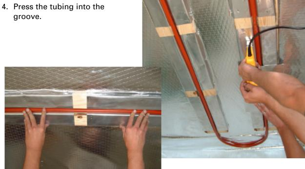
Staple some flat aluminum stock (unbent) over everything to hold the tubing up and increase heat conduction to the sheet rock
