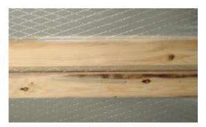
3. Then staple aluminum heat emission fins to the strapping. Use continuous covering with only short gaps.
