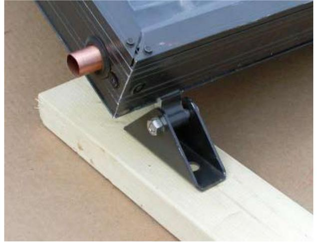
2. The front AE-Clips are attached to the front "Triangle Roof Mounting Brackets" with 3/8" x 1-3/4" SS bolts as shown in *Figure 5*.
