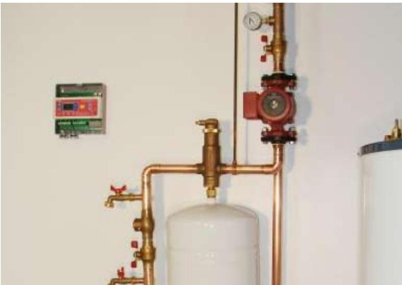
Locate these valves high and out of the reach of children and limit access to the mechanical area to adults. Attach caps and tighten very snugly with a wrench (more than hand tight) to discourage tampering.
