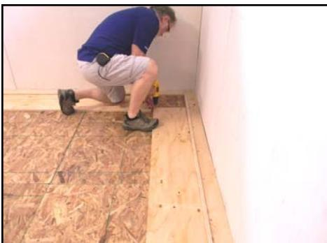
Using a piece of the ¾" plywood for a spacer, screw the strips down leaving a ¾" gap between them. At the end of the run where the tubing will turn 180 degrees, end the plywood strip about 12" away from the picture frame. This will allow for the tubing to bend and you'll fill in this area during a later step.
