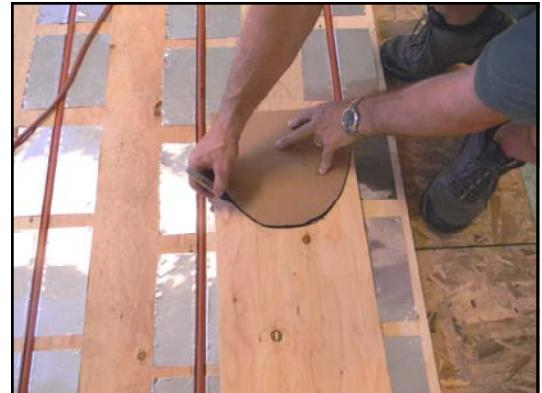
Take this piece of cardboard and place it down on a piece of plywood and trace it. Take a jig saw and cut around the half moon. Now take this piece of plywood and put it back in place on the inside of the tubing bend. To fill in the corners, follow the pictures below.
