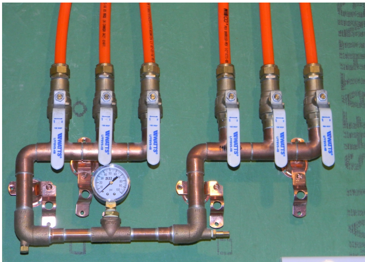
Wall-mounted manifold for zone located manifold or homeruns.
