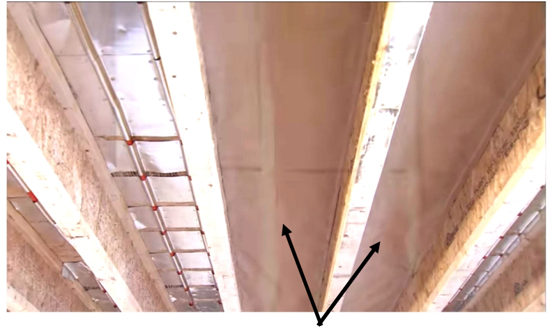
Reflective barrier installed
