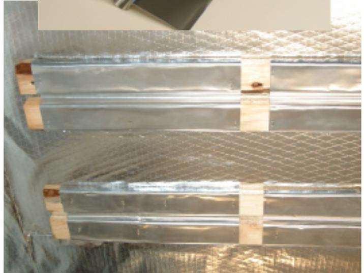
4. Press the tubing into the groove.
