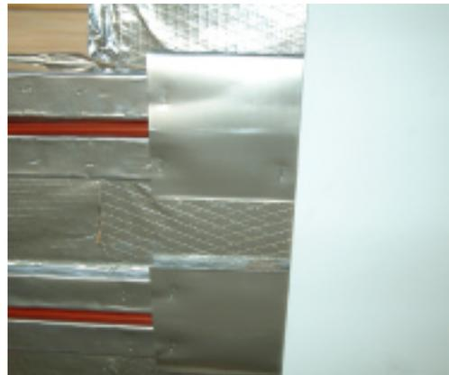
7. Run the tubing ends back to the water heater and control with the usual pumps and thermostats.
