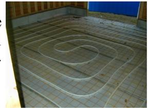
Instructions for installing tubing between the **floor joists**. If you have access to your floor joists from below then you can install radiant heat. This manual shows you how! Installation Supplement 260.
